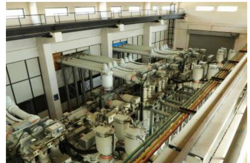
220kV/33kV GIS Substation, Dholera
