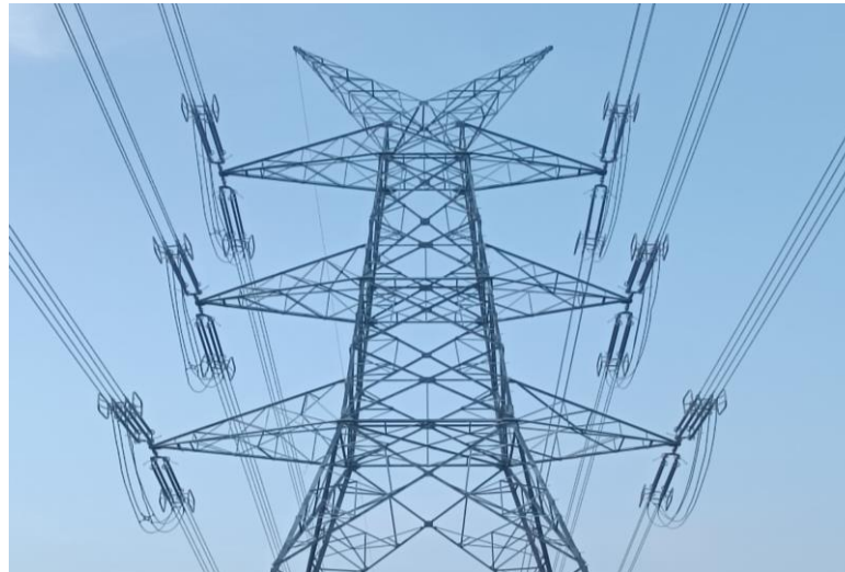
400kV D/c Transmission Line, Neemuch - Mandsaur
