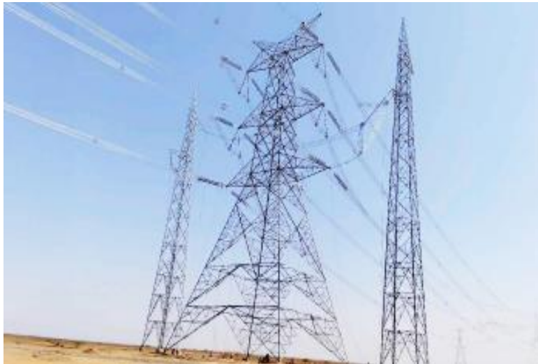
765 kV D/C Transmission lines in Khavda
